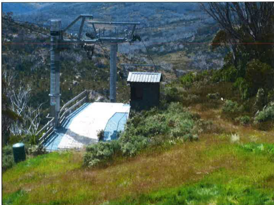
Photo 1 – Ridge Quad Chairlift midstation, view looking downslope
